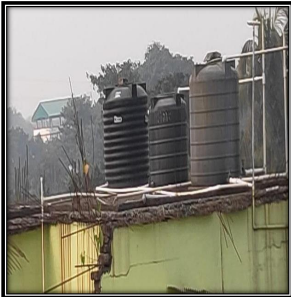
D. Water tanks on roof-top
