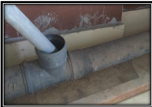
D. Drainage for liquid disposal
