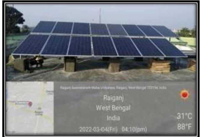
A., B. Installation of solar panels (15 nos) of 5kW power using RUSA 2.0 fund.
