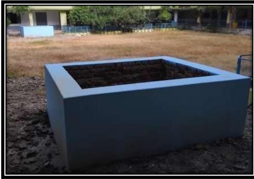
A. Tanks for storing rain-water (used for watering garden plants)
