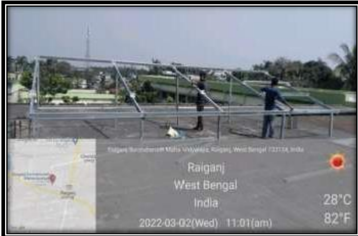
A., B. Installation of solar panels (15 nos) of 5kW power using RUSA 2.0 fund.
