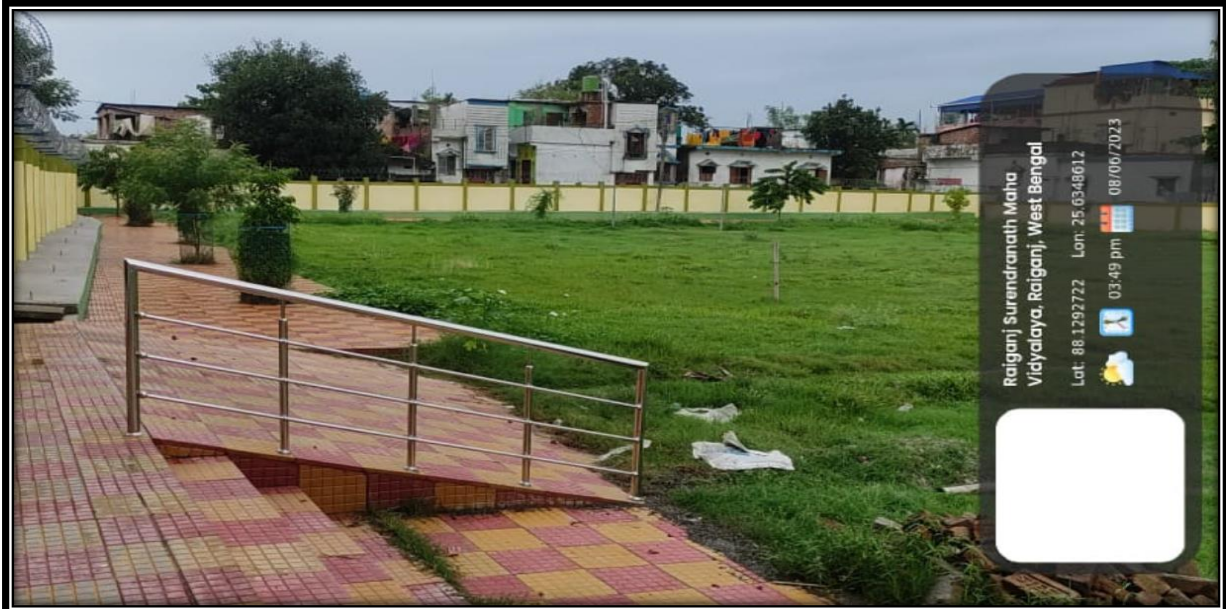
Ramp with railing for candidates with locomotory challenges
