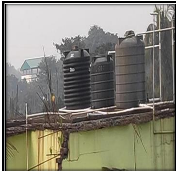
Construction of tanks
