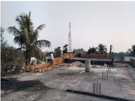
2 nd Floor Roof
