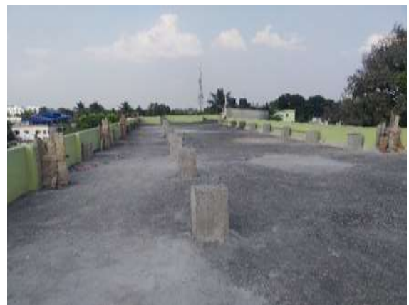
2 nd Floor Roof
