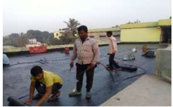
Picture after Renovation
